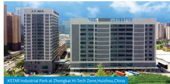
KSTAR Industrial Park at Zhongkai Hi-Tech Zone, Huizhou, China
